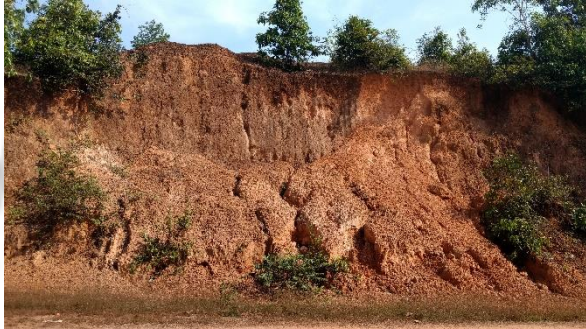
Photo: 6, Slides due to extensive cut slope in the study area.
